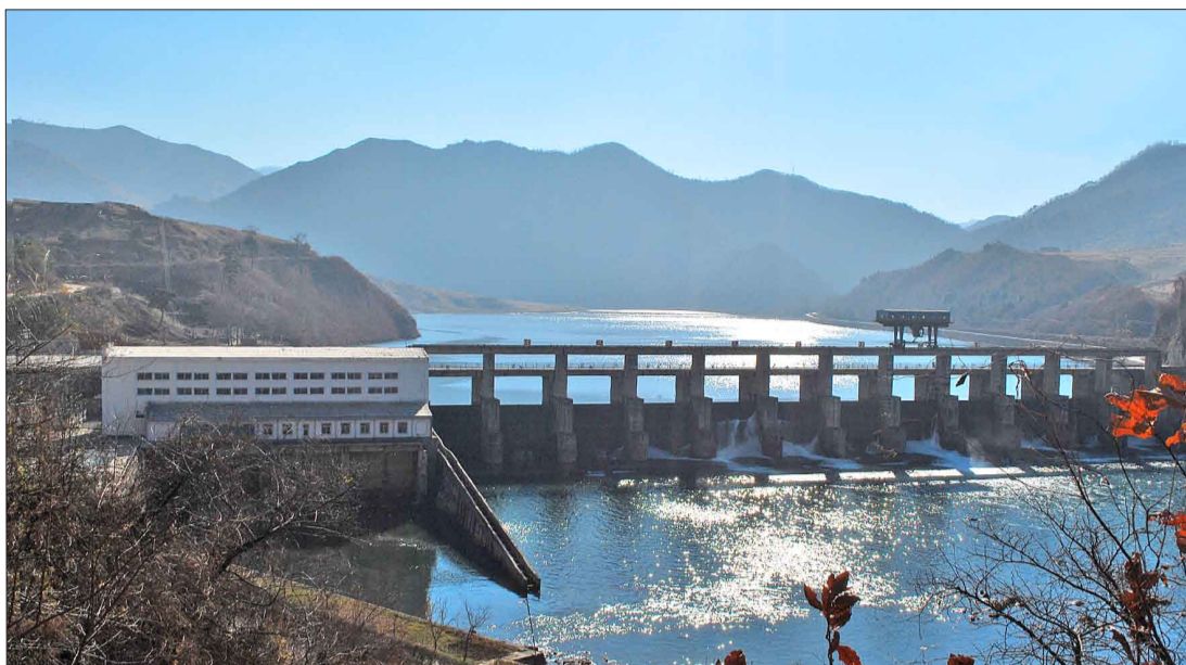
Power generation is on the increase at the locally-built power station.
