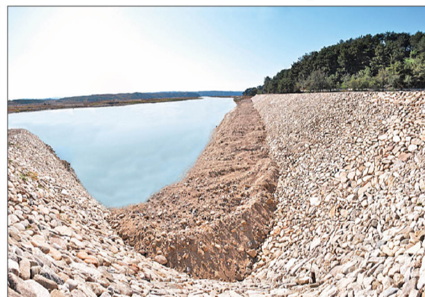
Part of rebuilt banks of the Kuryong River.
