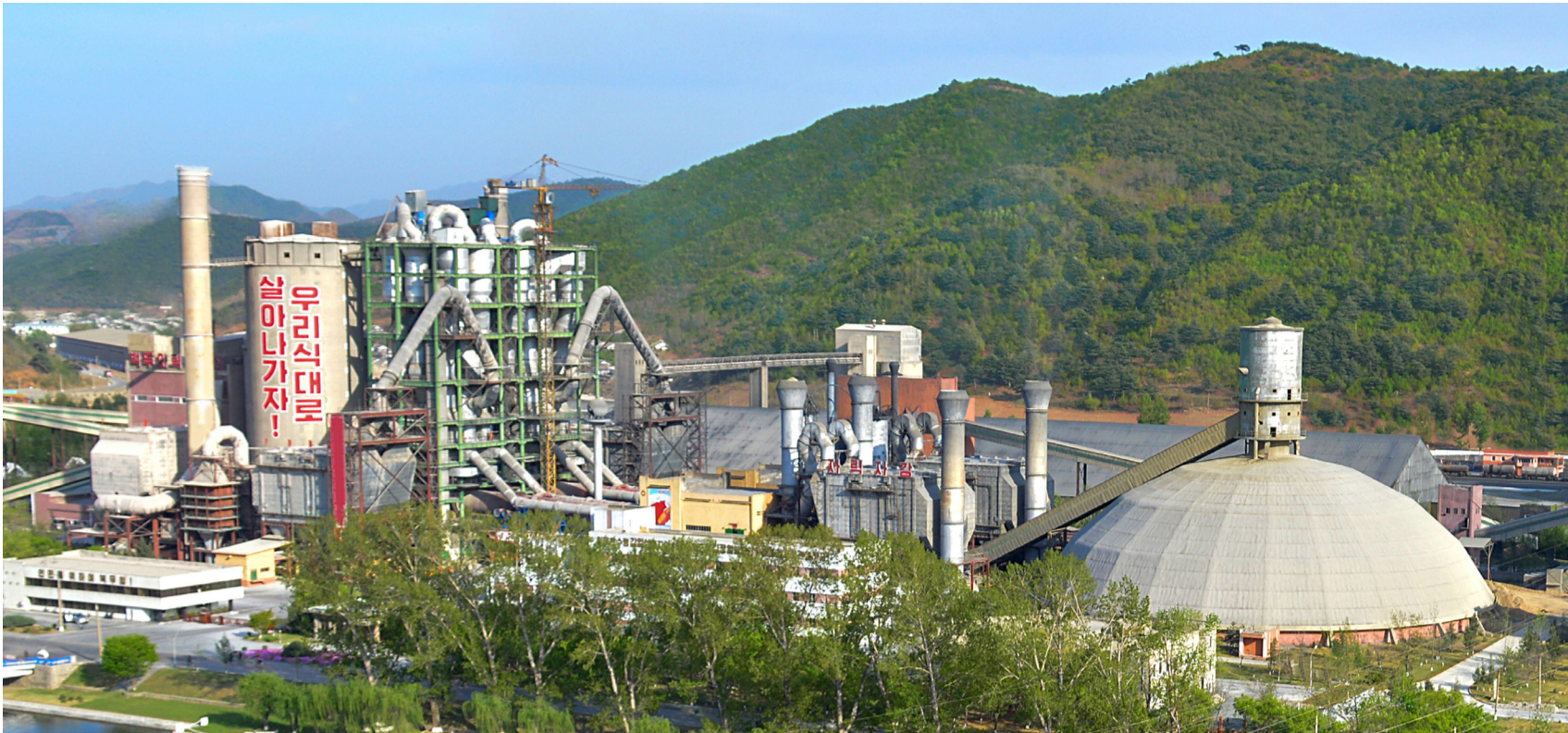
The Sangwon Cement Complex consists of the cement and refractory factories and a limestone mine. RYU KWANG HYOK / THE PYONGYANG TIMES
